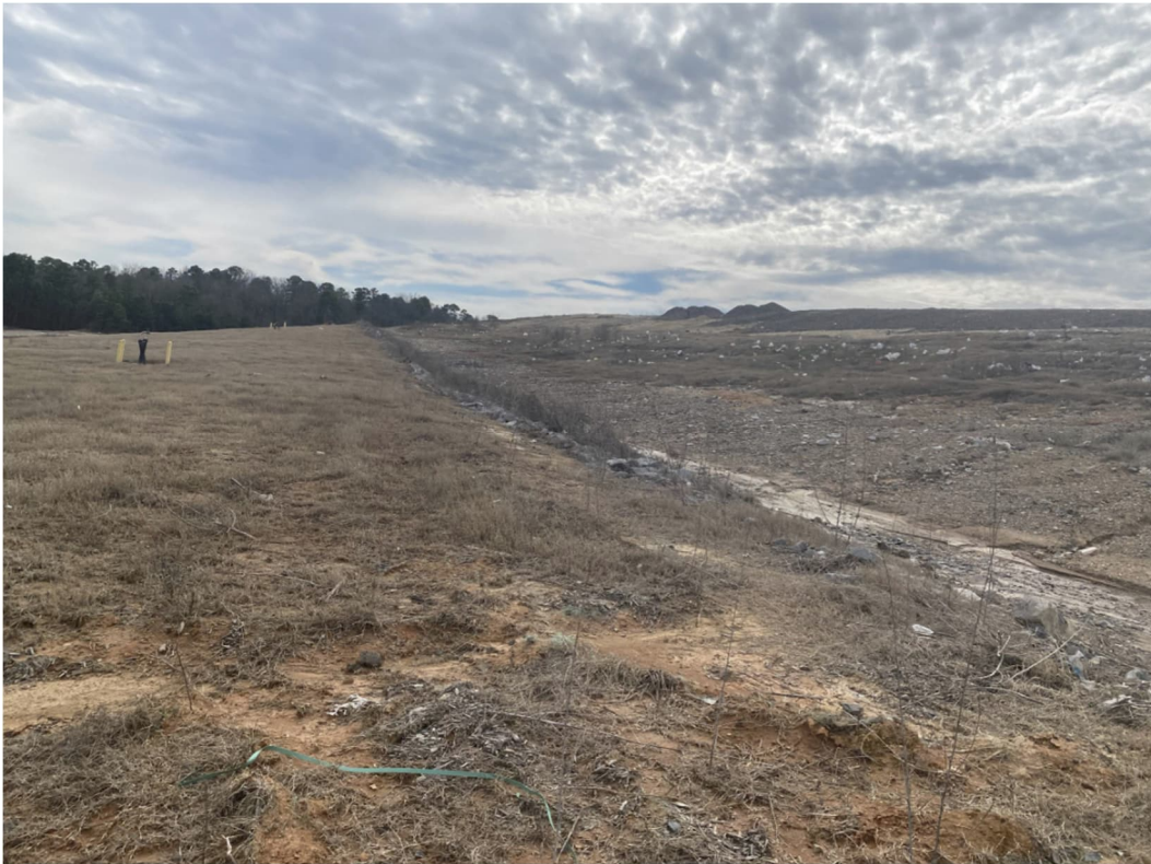
Looking south over east slope of Cell 4
