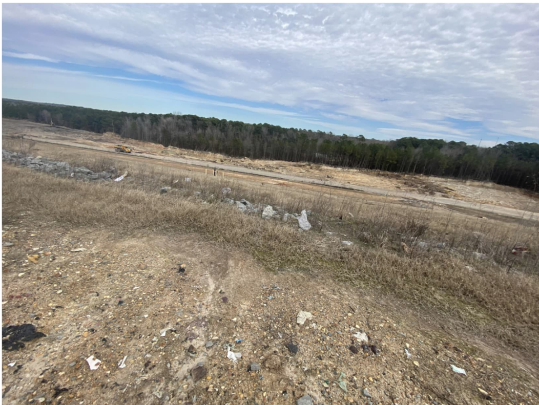
Looking east over east slope of Cell 4
